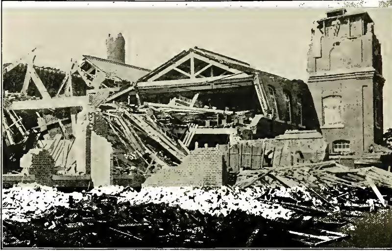
FIG. 284. — This building was torn in pieces by the shaking of the earth during one of the destructive Japanese earthquakes.
